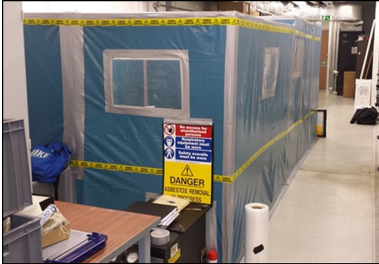
Fig. 8. Asbestos enclosure erected within storage area at National Museum Scotland.
