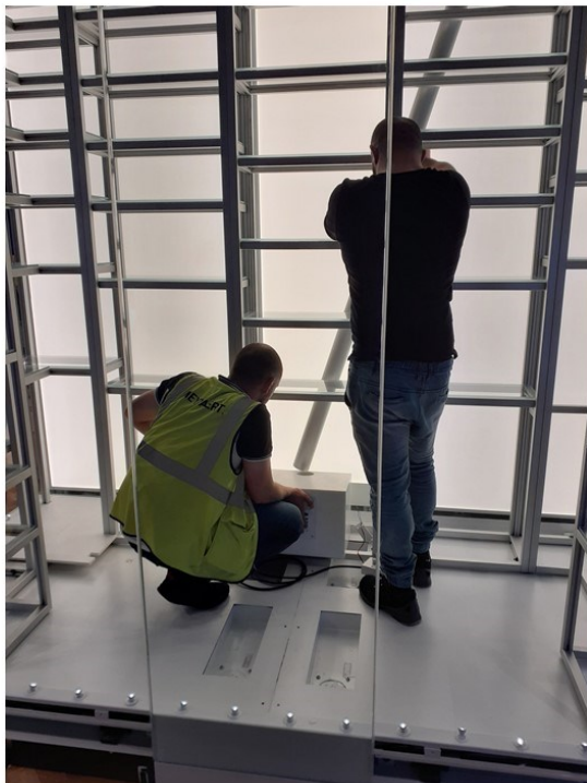
Figure 7. The instillation of the aluminium frame carried out by staff from Meyvaert, with the completed shelves for the back and side of the case. (Photo Jan Freedman)
