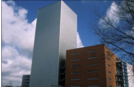
20 floors of purpose-built collections' storage
